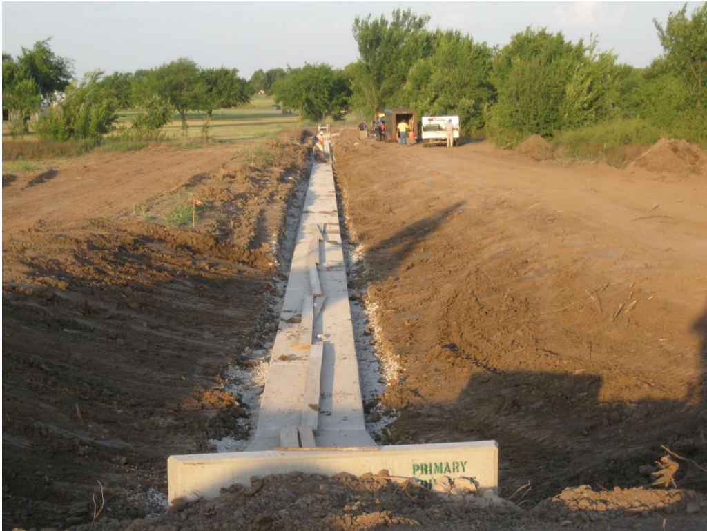
Work on concrete lined ditch channel for Phase 2
